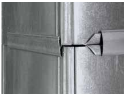
„S“ seam and drive cleat
