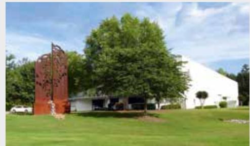
RAS Systems LLC in Georgia, USA
