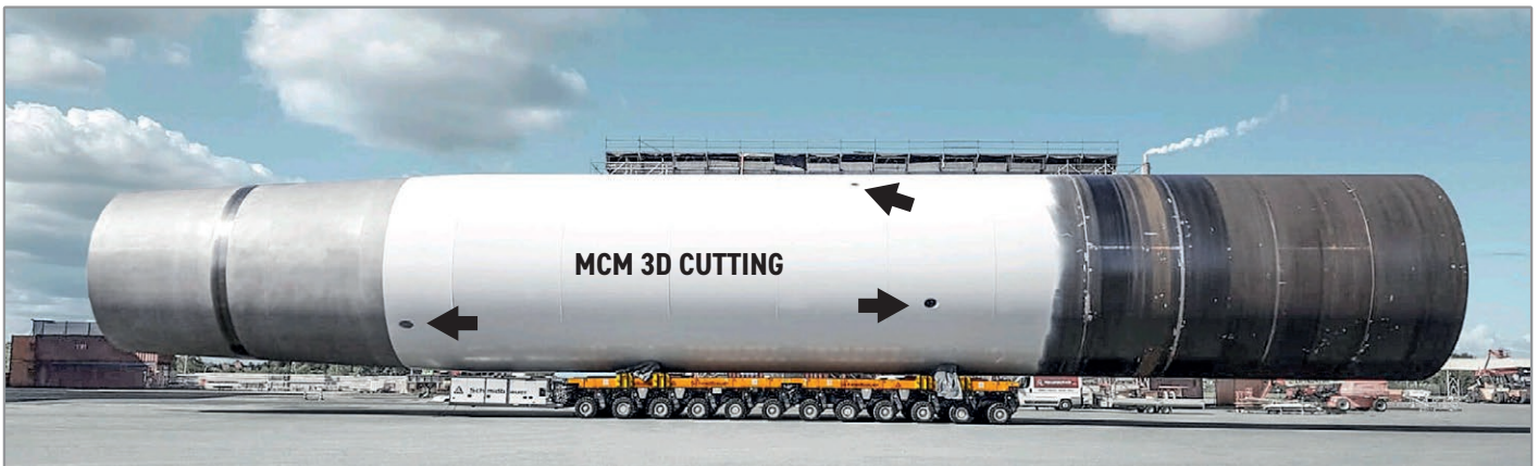
Overall view of XXL monopile
