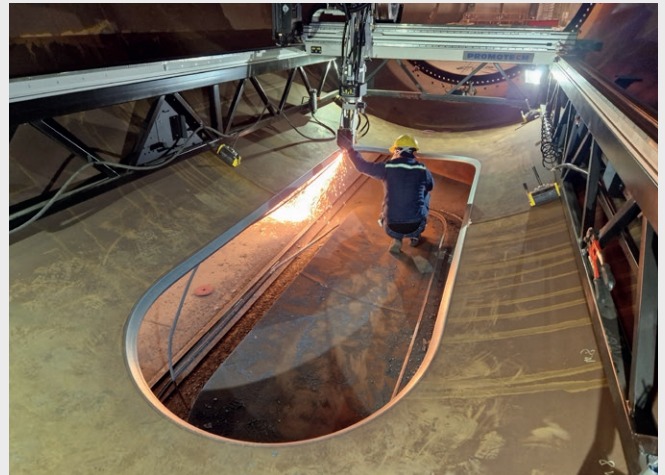
3D CUTTING & WELDING (SAW)
